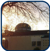
Trollhatten renovation project
