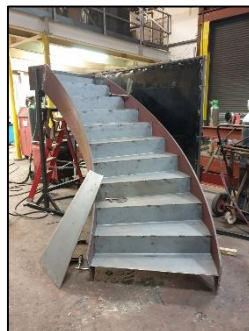
Stairs being built
